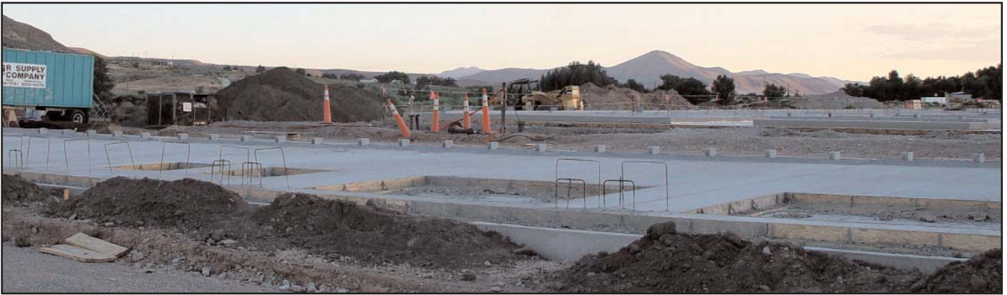
This new geo-powered industrial park is currently under construction in Elko
